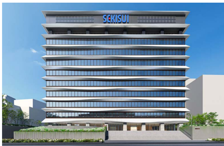
Conceptual diagram of the Group's Osaka headquarters after completion of renewal work.
